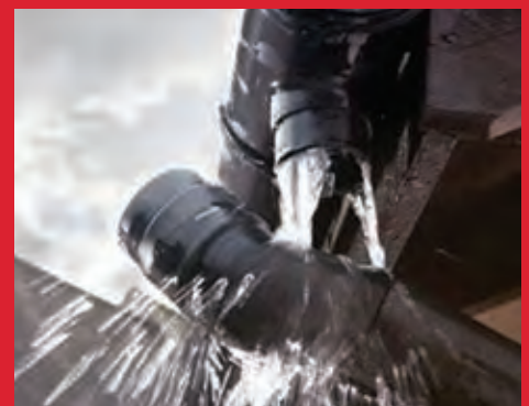
Plumbing systems and suspended pipes
