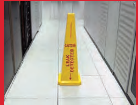
Raised floor computer facility
