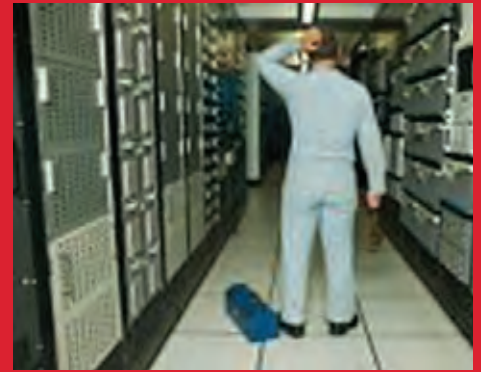
Server and communications facility
